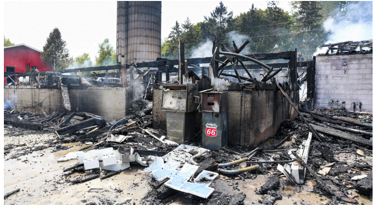
Barn Fire on Rose Farm Road - 07/01/2024
